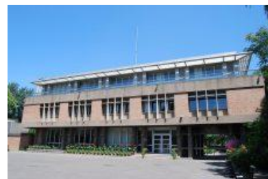
Embassy office building
