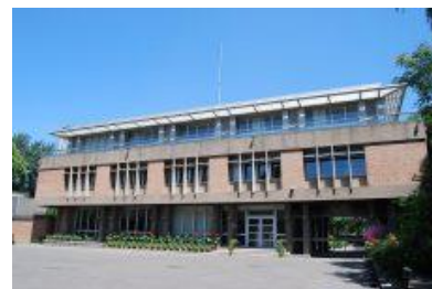
Embassy office building
