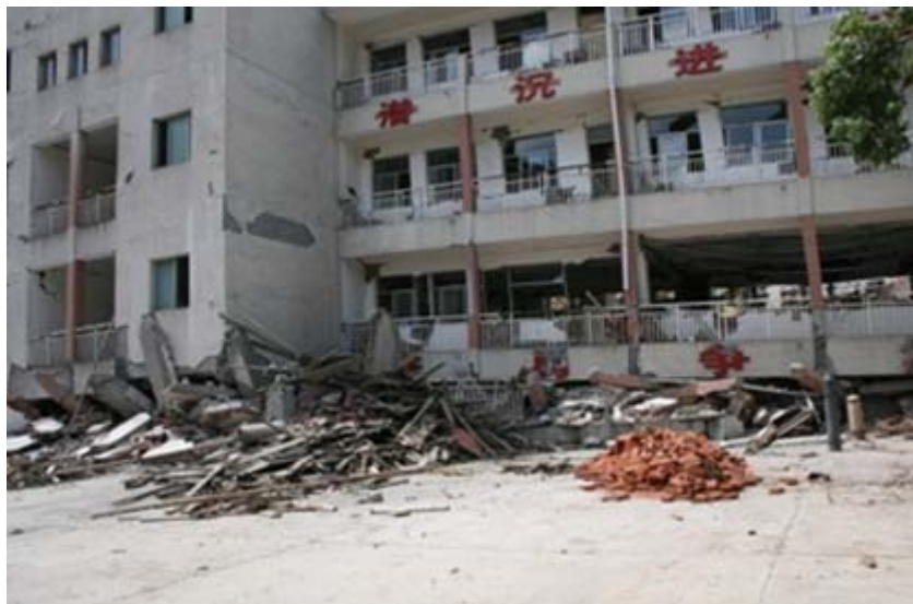
A collapsed school building in Beichuan county (International Federation).
