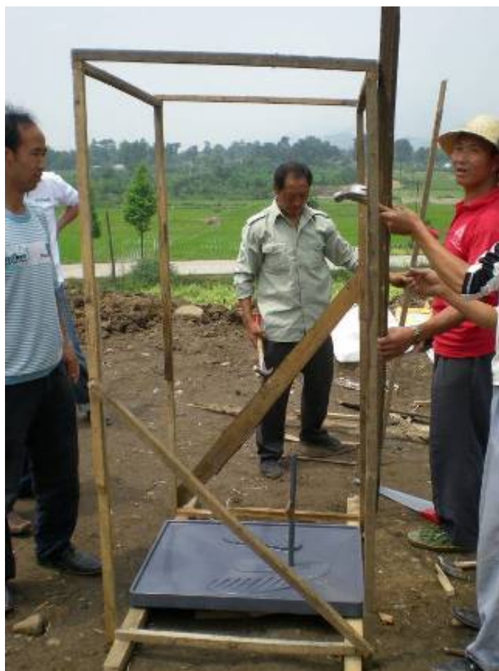
Members of the community gather around to set up their own latrines. International Federation.
