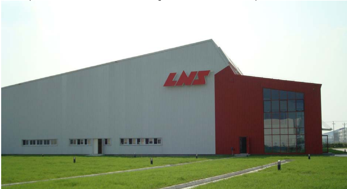
Legend: The new production plant of LNS SA in Wujiang.
