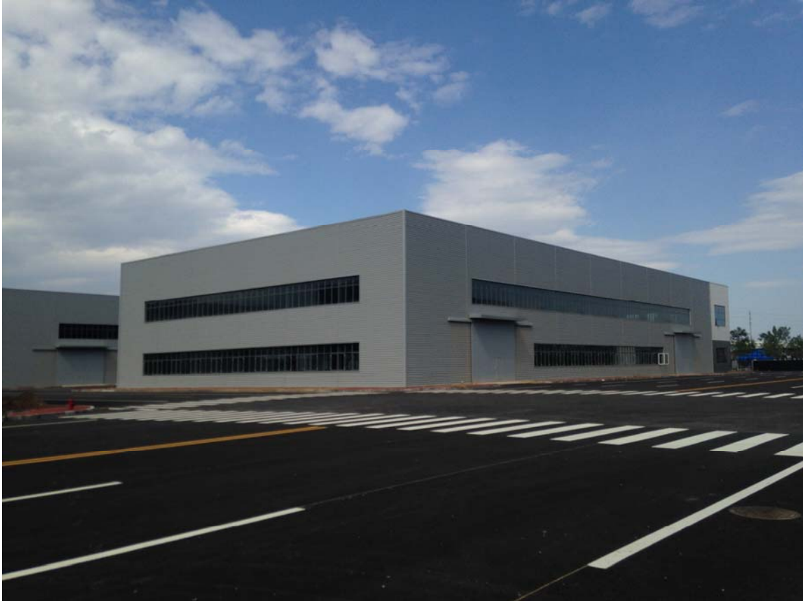
Picture legend: In the Wuqing Industrial Park, the Swiss Center Tianjin offers first class workshop and assembly space for Swiss companies. (Picture source: swisscenters.org )
