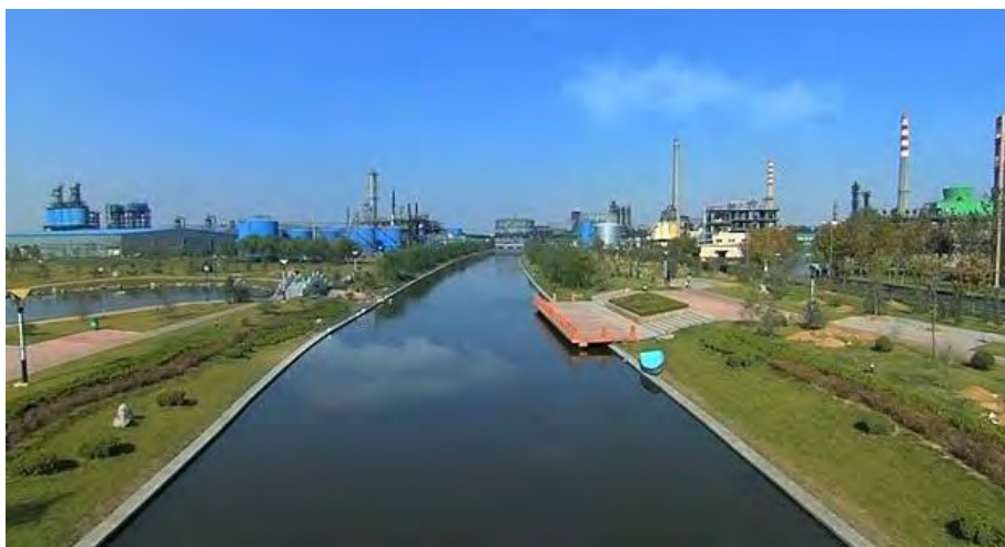
Site of the planned propane dehydrogenation unit in Qingdao, China. (Photo: © Jinneng Science & Technology Company, Limited)
