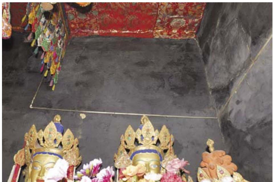
(Fig. 4) Back wall of the principal shrine showing area to be restored (Photography by Luigi Fieni)
