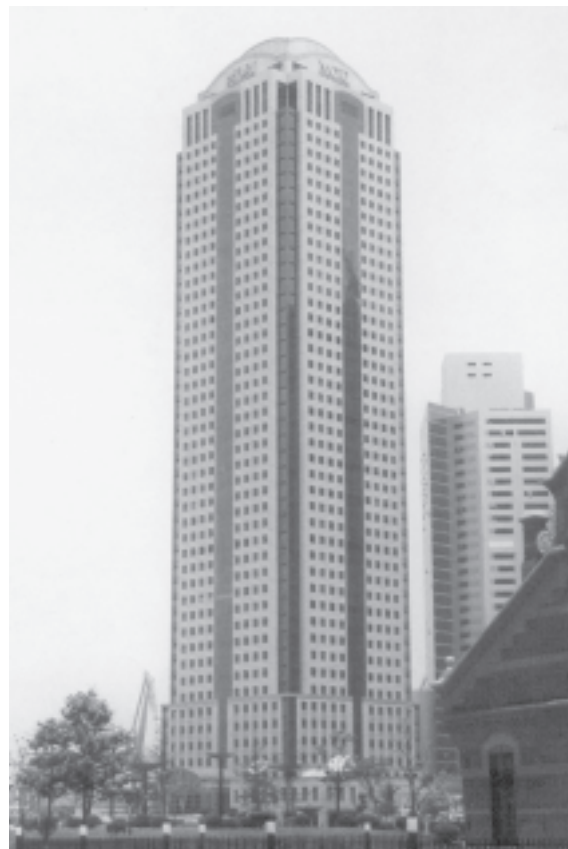
The HSBC Tower in Shanghai.
